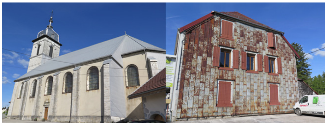
Church with zinc cladding and building with galvanized iron cladding in Mouthe, France
